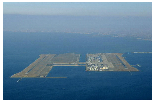
Figure 4 Overview of the airport.
