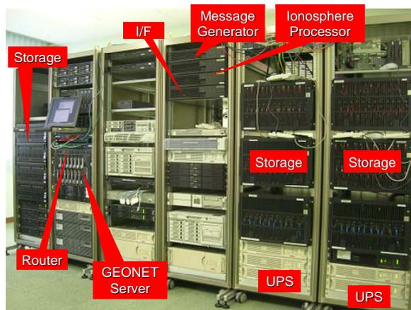
Figure3 L1-SAIF Master Station (L1SMS)
