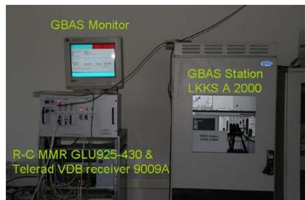
Fig. 1: GBAS ground station and monitor installation
