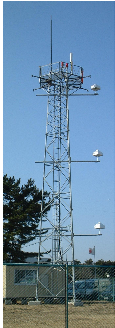
Figure 7: New VDB stacked array antenna Height of segment was 15.5m (top), 10.5m (middle), 5.5m (bottom) each. Another GPS antenna for kinematic reference was mounted on top of this tower, height of 17.2m.
